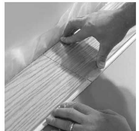
6. Drop second board into place ensuring that the seam is tight.
