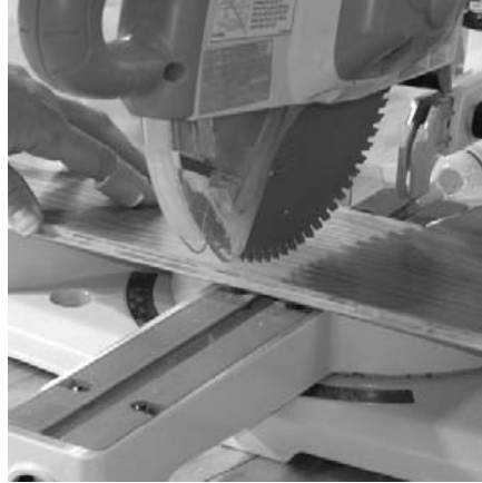
8. The cut board from the first row is used to start the second row.
