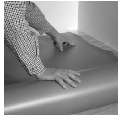
3. Roll out the underlayment, a few rows at a time to prevent tearing.
