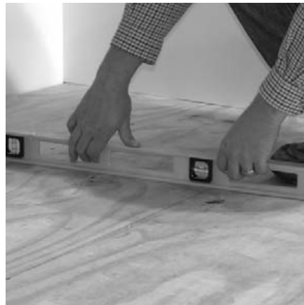
2. Make sure the floor is level and dry.
