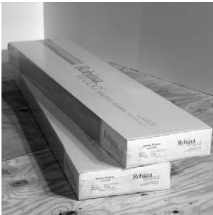
1. Allow flooring to acclimate to the installation room's temperature.
