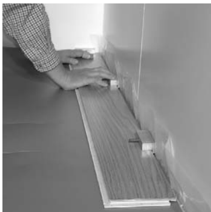
4. Start in corner positioning first board with 1/2" expansion spacers.
