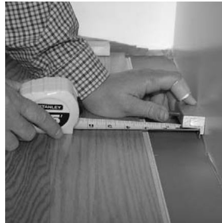
11 Measure cut line for last row, allowing for 1/2" expansion.
