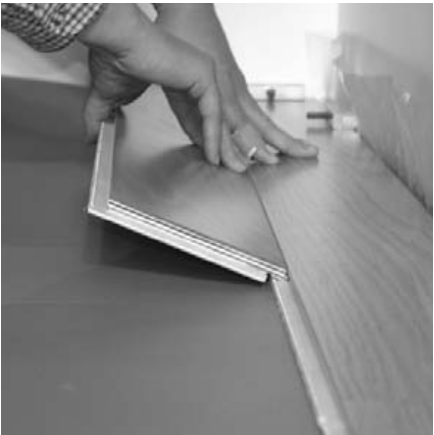
10. Position second row board at an angle and push down into place.
