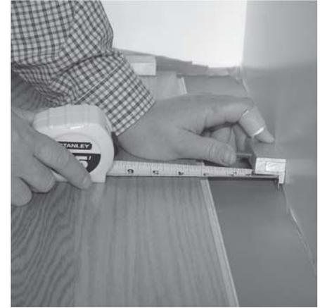
12. Measure cut line for last row, allowing for 1/2" expansion.
